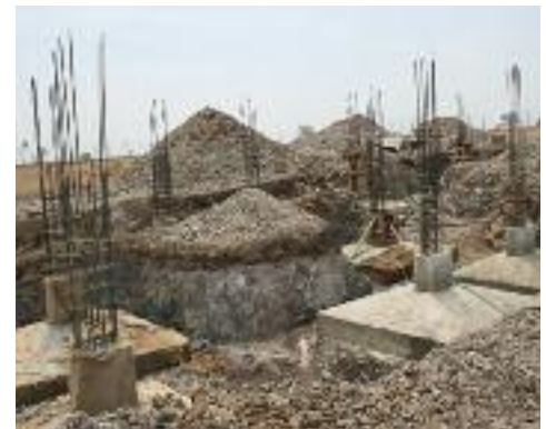
School footings poured
